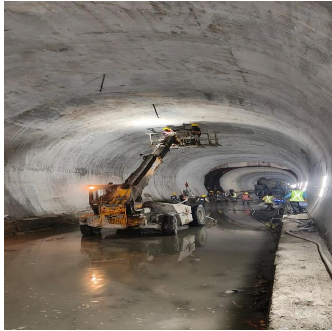
Fig.3. Tunnel Excavation and Lining Works During Construction.
